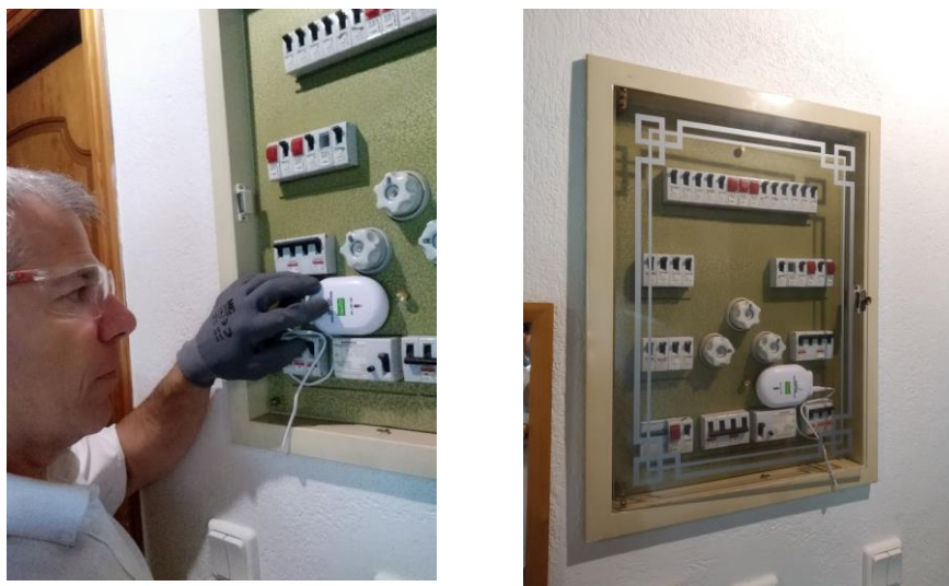
Figure 12: Installation of electricity consumption meters
